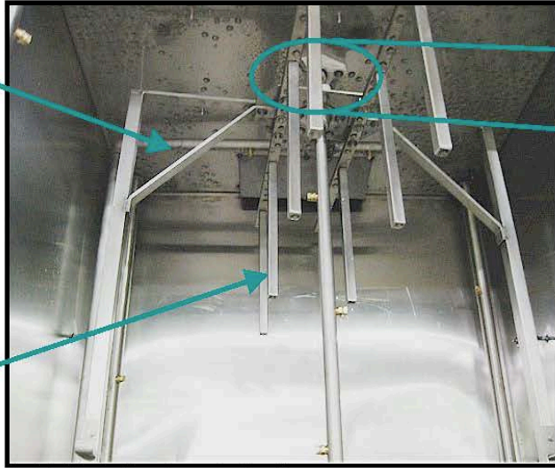
Inside Wash Chamber – Ceiling View
